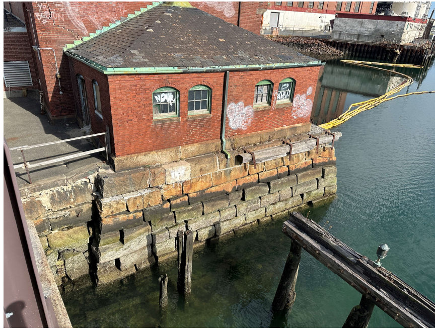
Figure 4: View of South Wall from Alford Street Bridge
