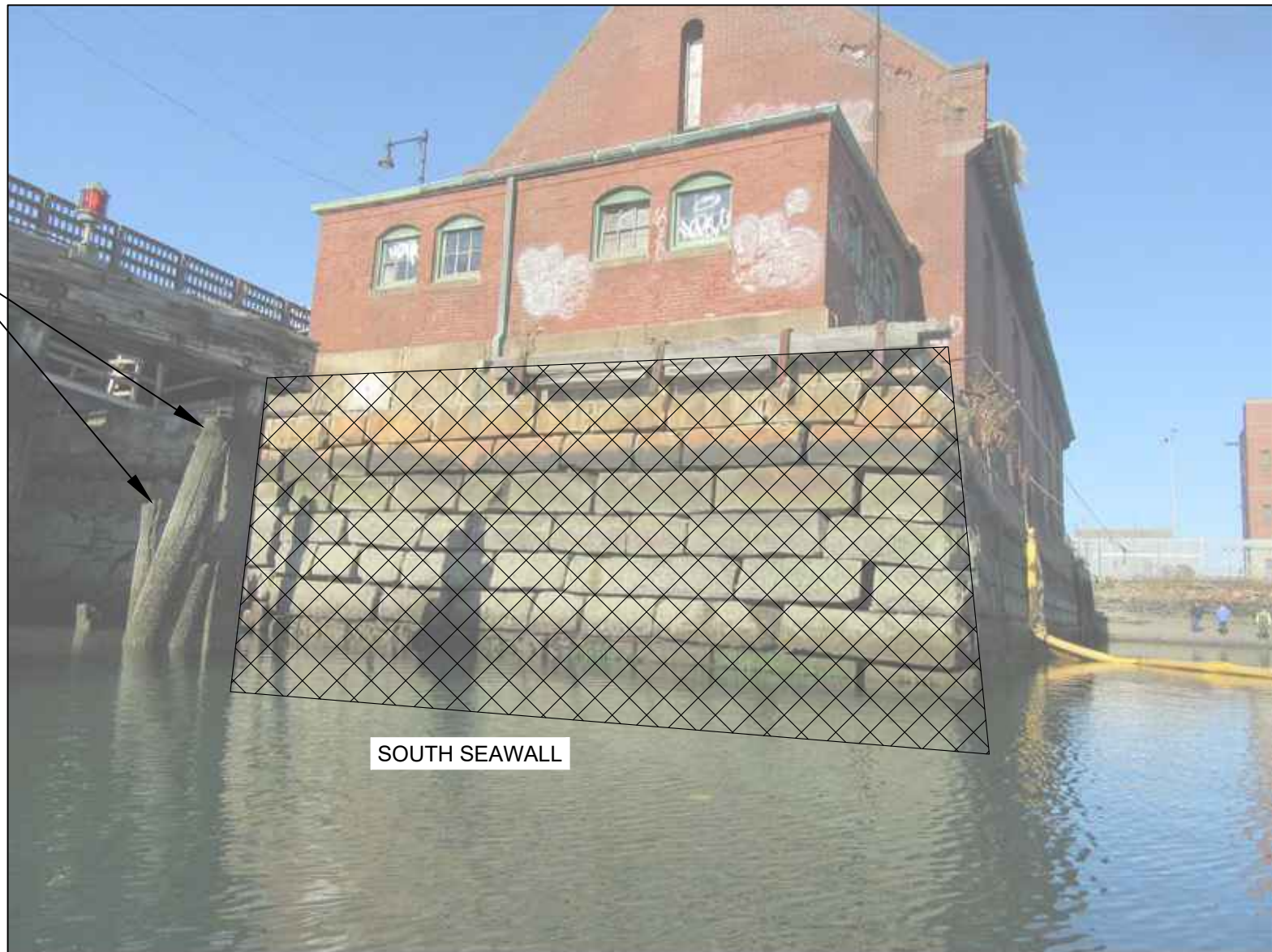
PHOTO 10: EXTENTS OF SOUTH SEAWALL STABILIZATION
