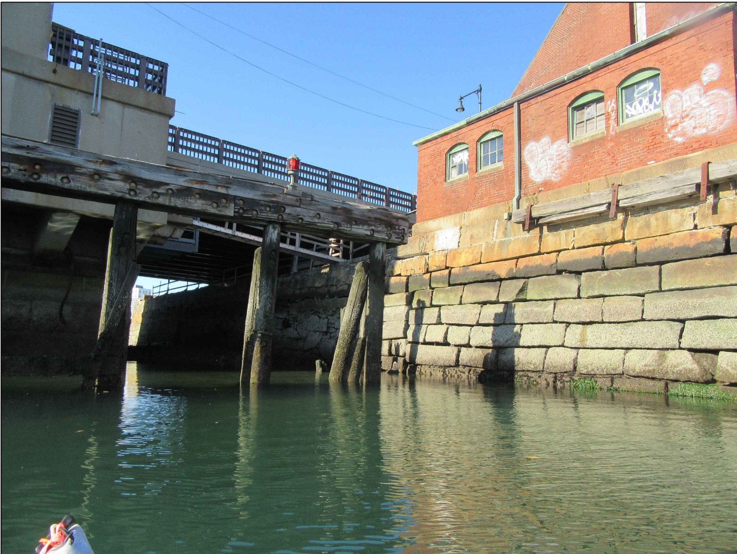
PHOTO 9: TIMBER BRIDGE FENDER PILES ADJACENT TO SOUTH SEAWALL
