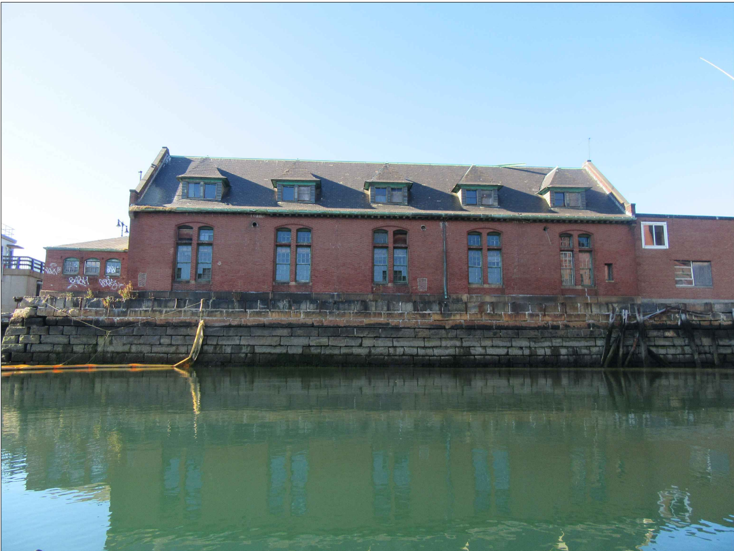
PHOTO 2 : EAST SEAWALL, LOW TIDE
