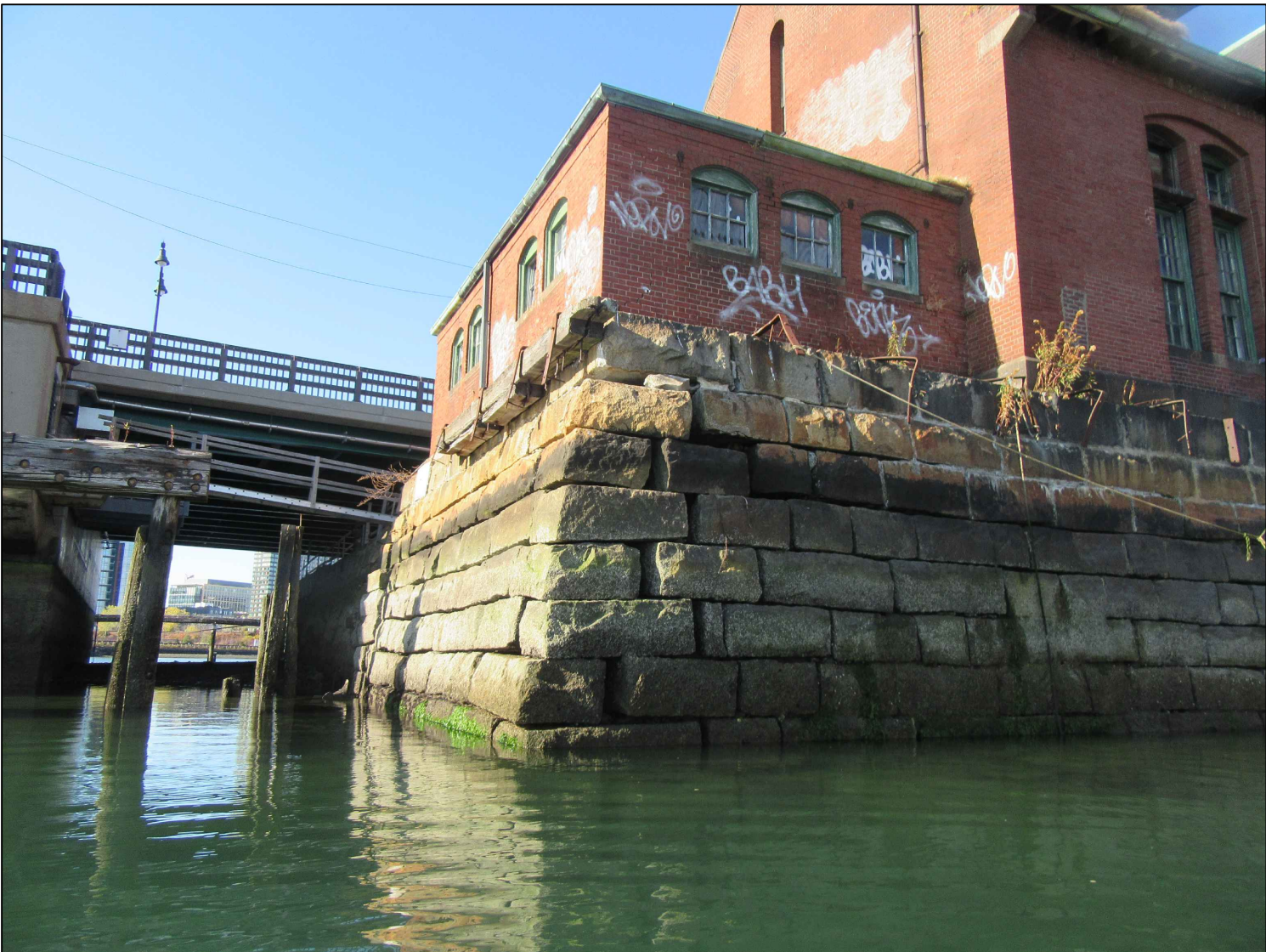
PHOTO 8: CORNER OF SOUTH AND EAST SEAWALL, LOW TIDE
