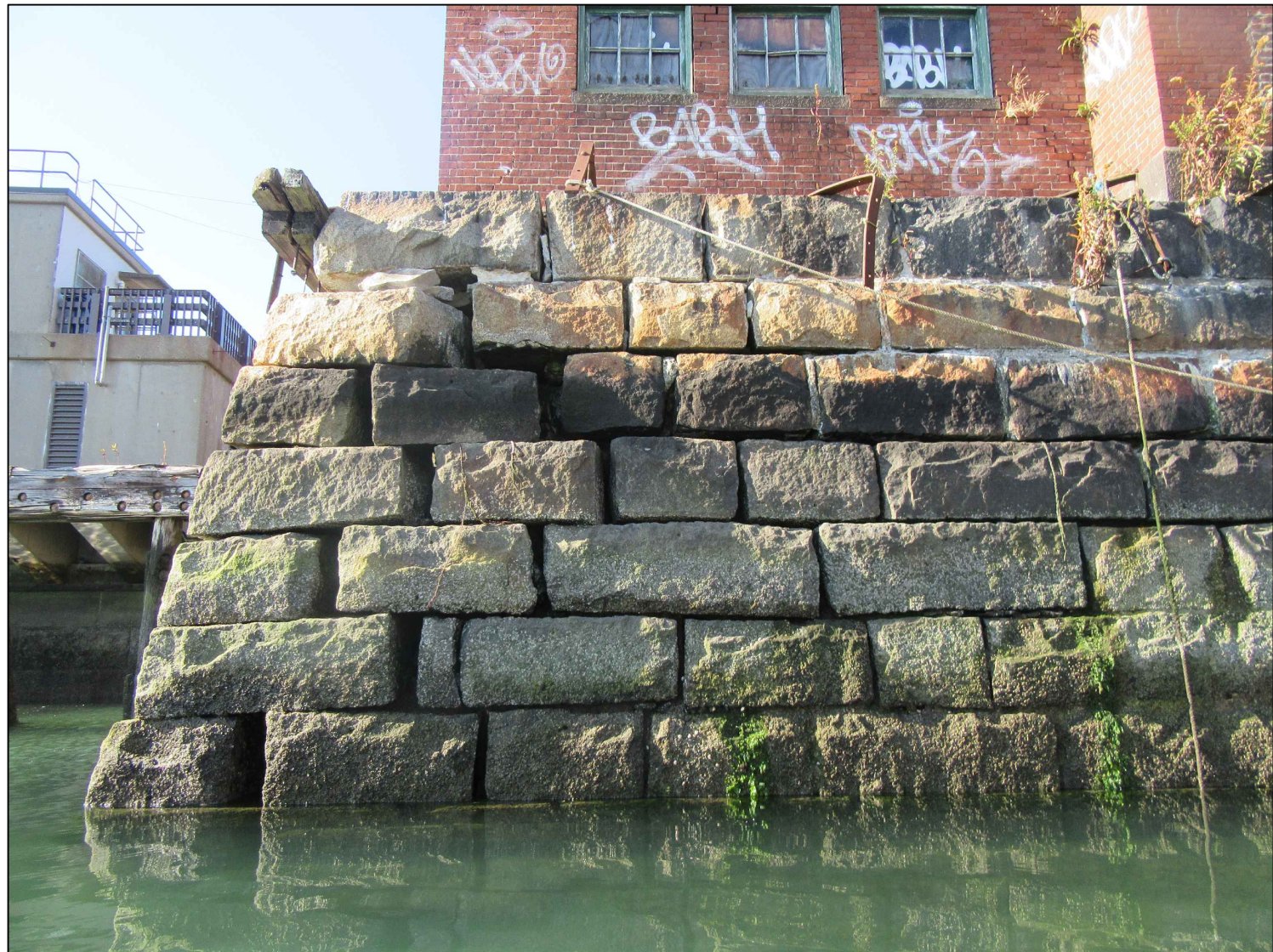
PHOTO 7: EAST SEAWALL, LOW TIDE
